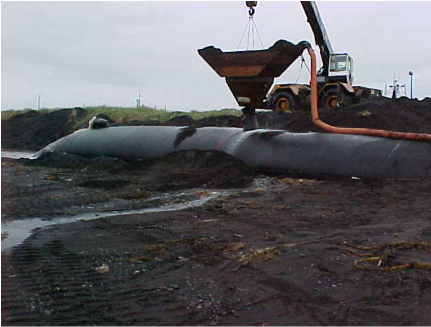
Photo 1: Demonstration Erosion Control Project; installation of geotubes, September 2005.
