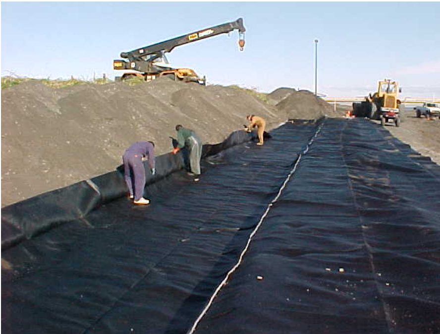
Photo 2: Community members preparing to install geotube near dock, September 2005.
